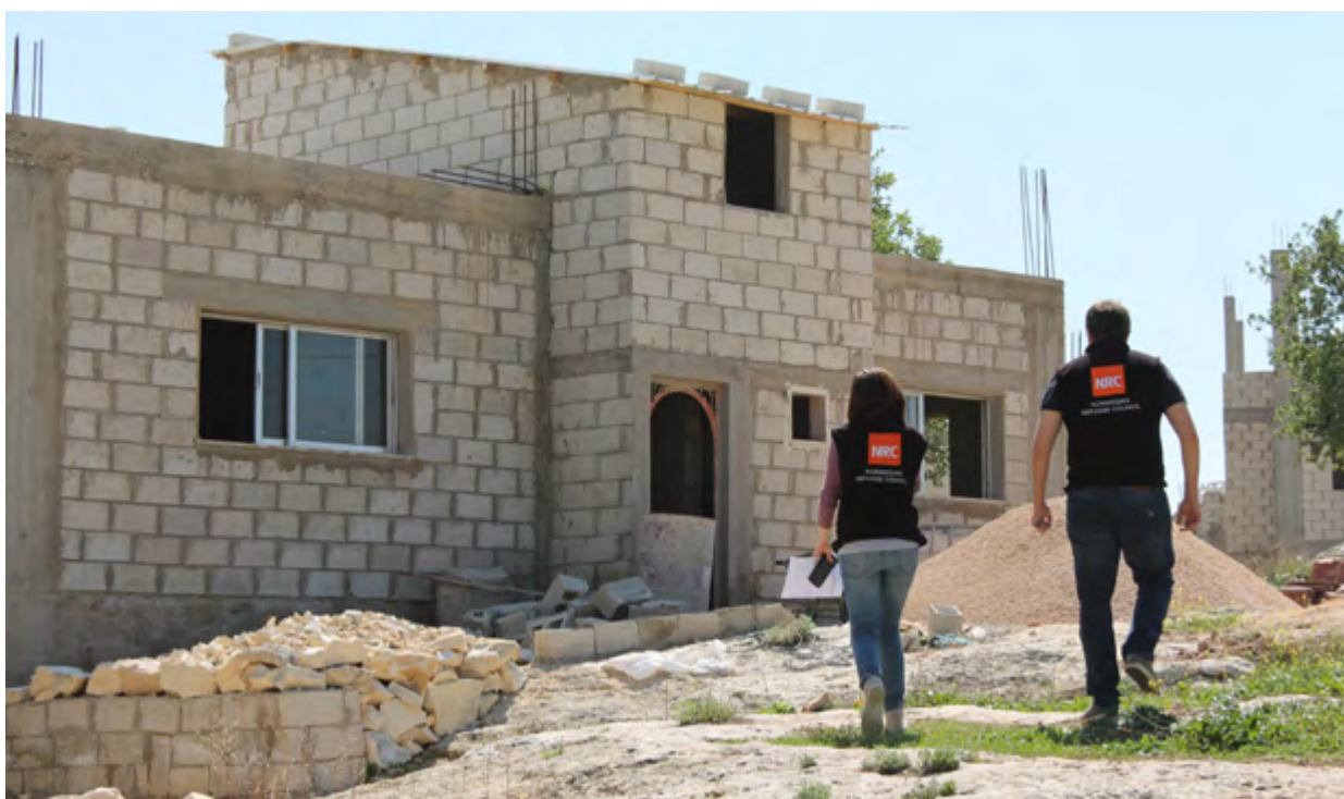
NRC engineers assess construction works for Syrian urban refugees in Jordan. Photo: NRC Jordan/Rawan Baybars, March 2014
