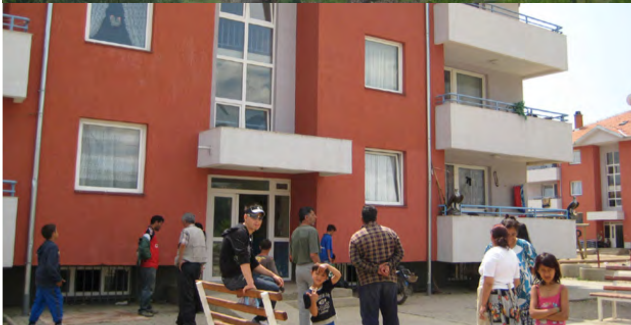
View of the destruction of Roma Mahalla after the conflict, and of a rehabilitated building. Photo: IDMC/B. McCallin, May 2009
