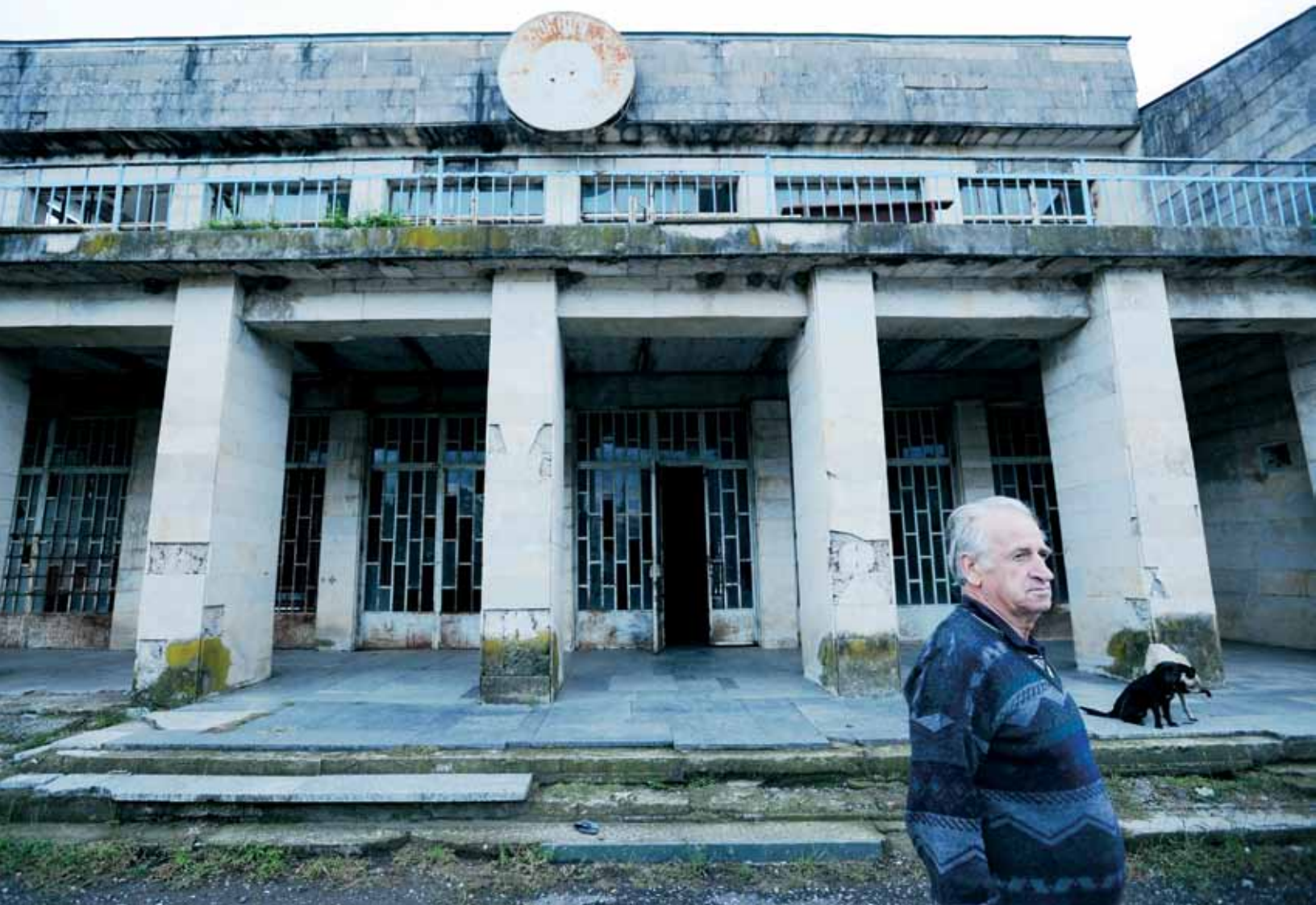
Revaz, aged 73, stands in front of the Khobi Swimming Complex, which has been a “collective center” for IDPs from Abkhazia since the conflict in the 1990s. The building is structurally unsound, has no running water and no functioning heating during the winter. Photo: UNHCR/ P. Taggart / October 2008
