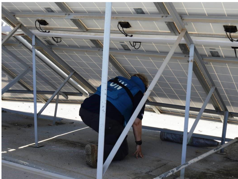
UNMAS risk assessment at Beit Hanoun Elementary School – photo credit UNMAS/Ahmed Joha
