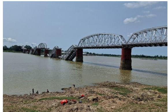
The March 28, 2025 earthquake caused widespread destruction to homes, property, and infrastructure, as seen by this bridge in Mandalay.
